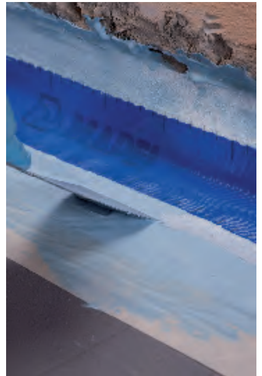
Application of Mapeband to a wall-floor joint with Mapelastiac AquaDefense
