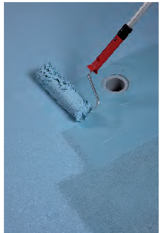
Application of the second coat of Mapelastiac AquaDefense
