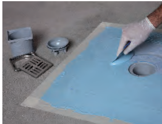
Impregnating Drain Vertical fabric with Mapelastiac AquaDefense
