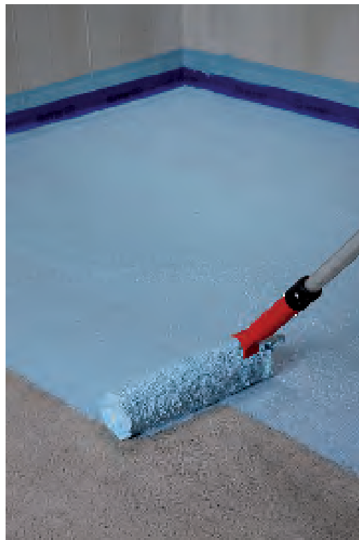
Application of the first coat of Mapelastiac AquaDefense
