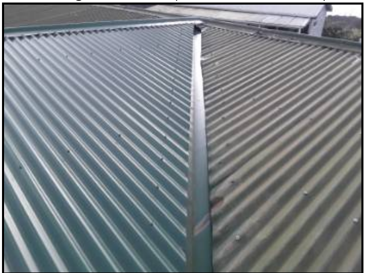
Valleys clear of debris.
