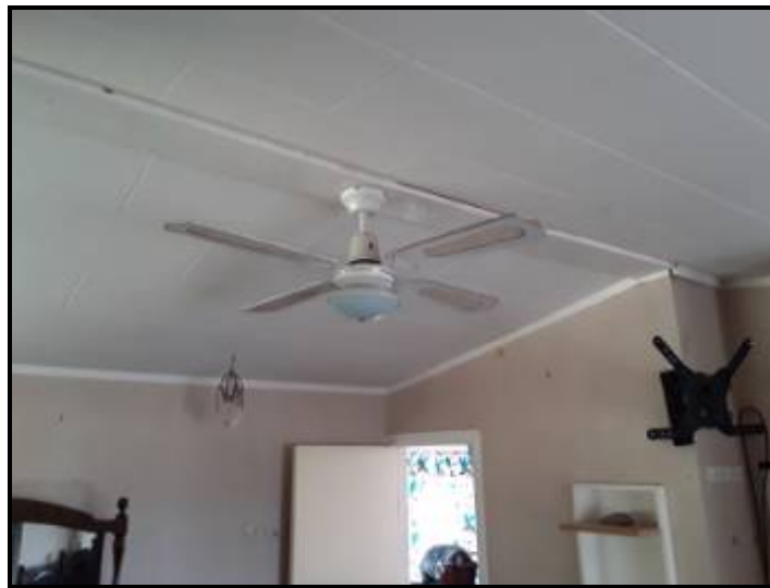
Bedroom ceiling tested dry at time of inspection.
