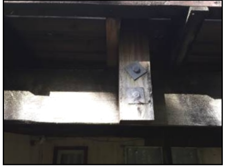
Solid bolting to handrail posts.
