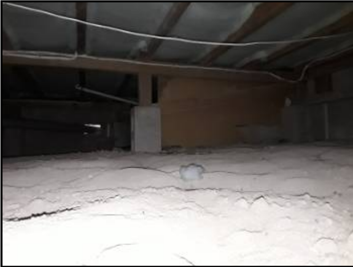
Posts and structural timbers appear solid.
