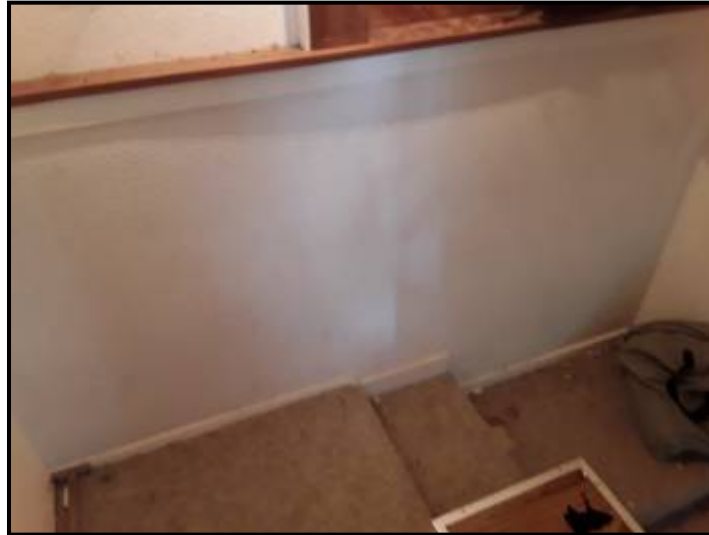
Missing handrail.
