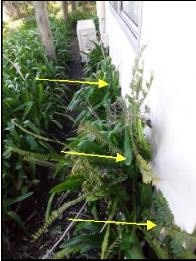
Cladding needs to ventilate to stay dry.
