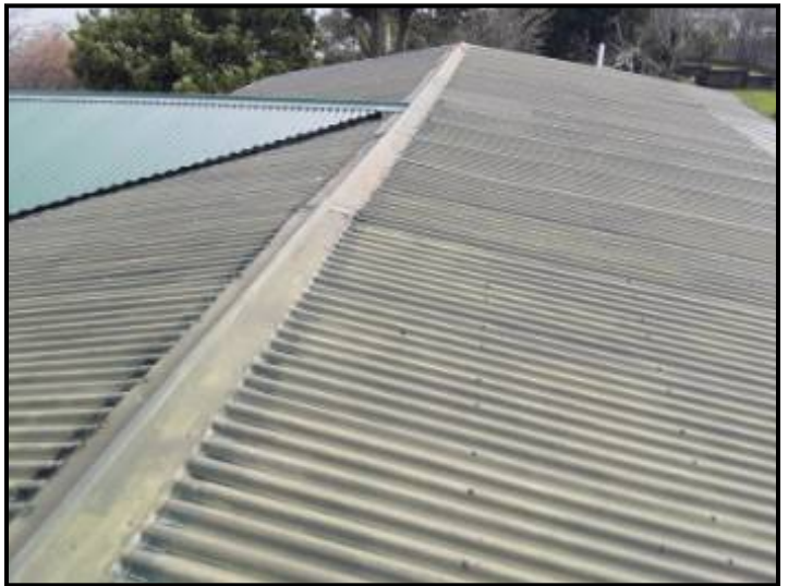
Roofing iron is in acceptable condition mostly.
