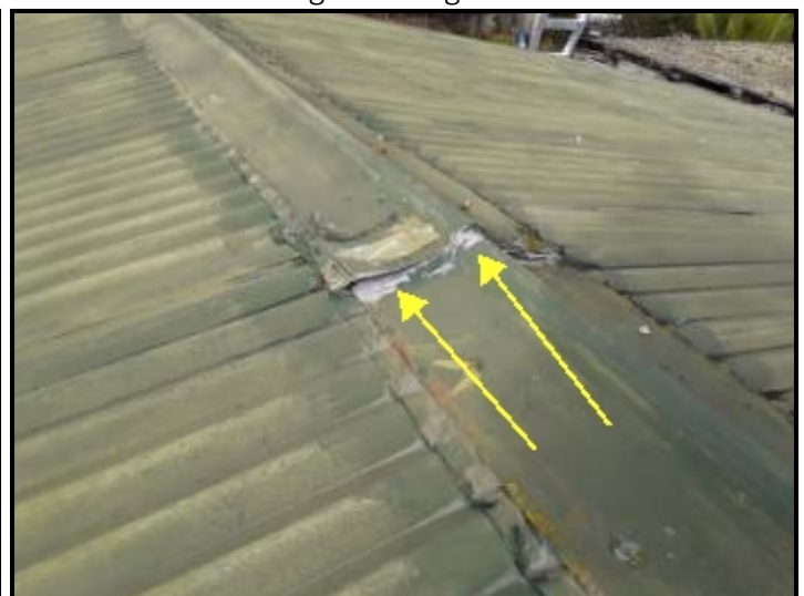
No seal to ridge cap joins.
