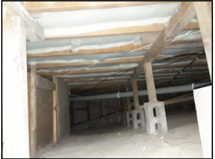
Insulation well installed.
