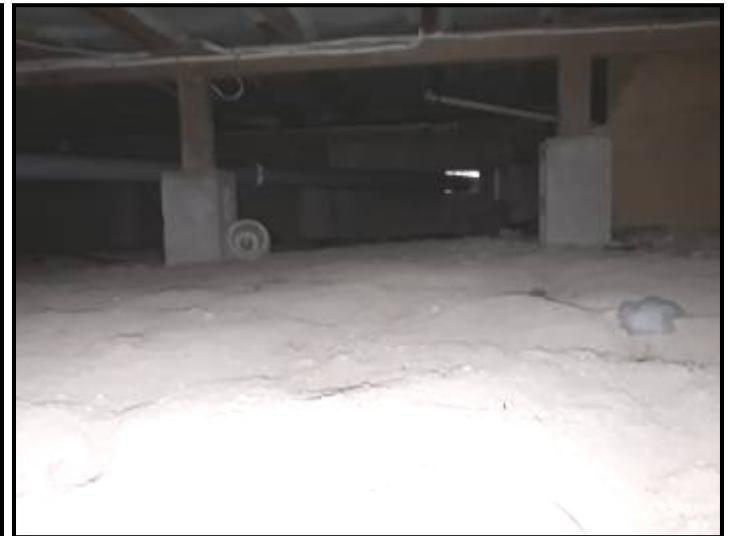
Structural timbers appear solid.
