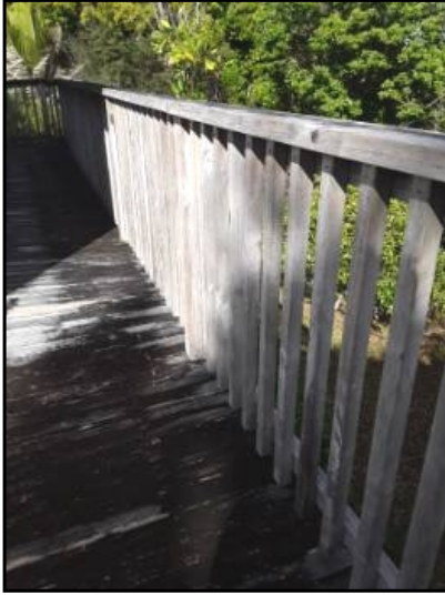
Handrails solid construction.
