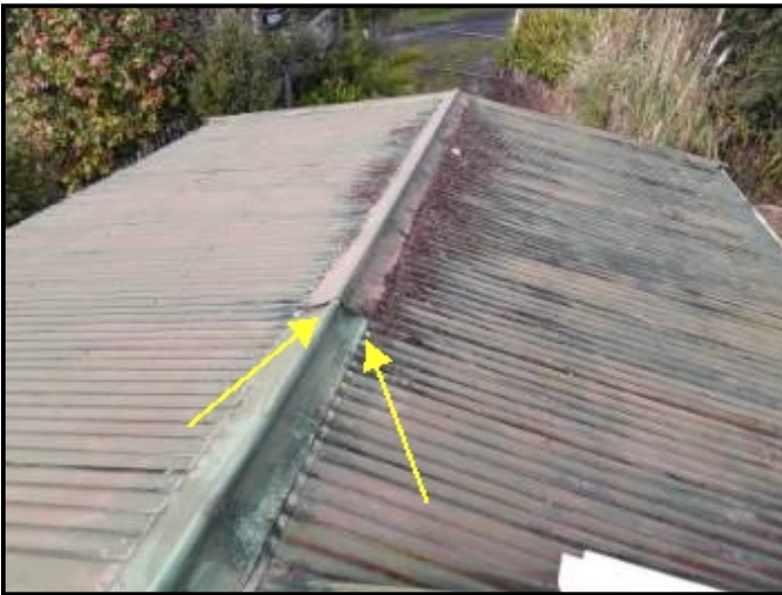
Garage roof same as main house roof
