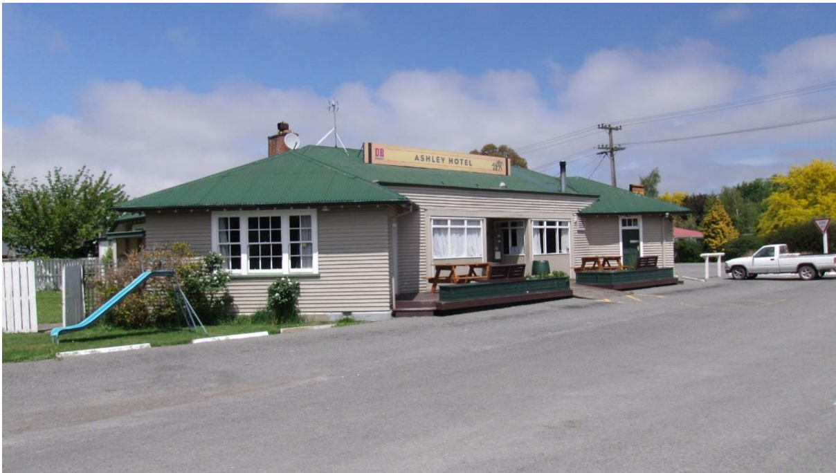
Photo 1. Ashley Hotel north-west elevation from Canterbury St.
