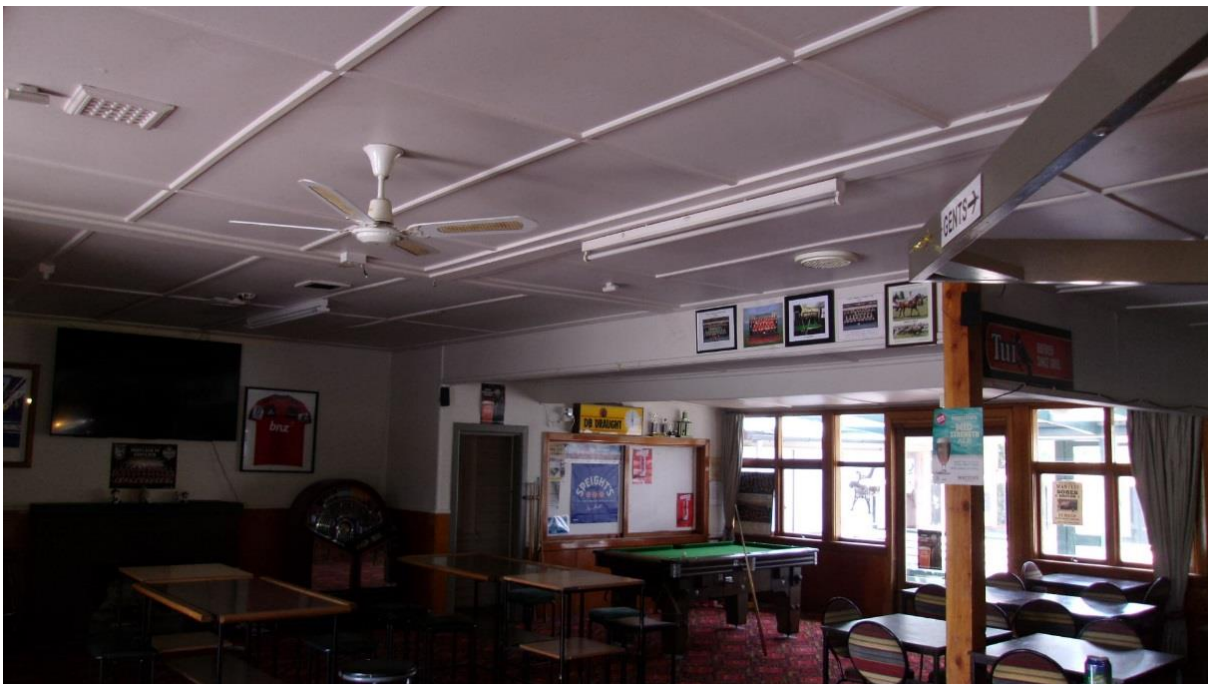
Photo 6. Interior of bar looking diagonally towards the east. (Fire place for one of double chimney at left). Pinex soft board lined walls and ceiling. Beams (unknown material) support roof over open plan bar area.
