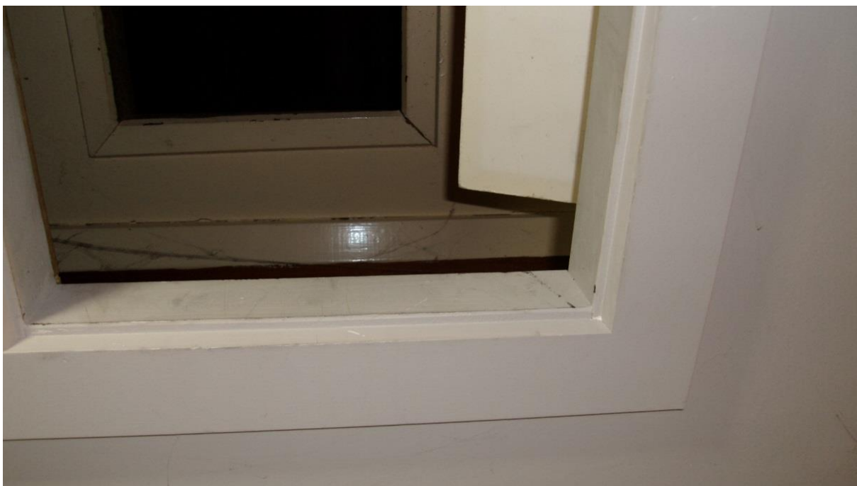
Photo 8. Hatches in the false and original ceilings in the Ladies toilet.
