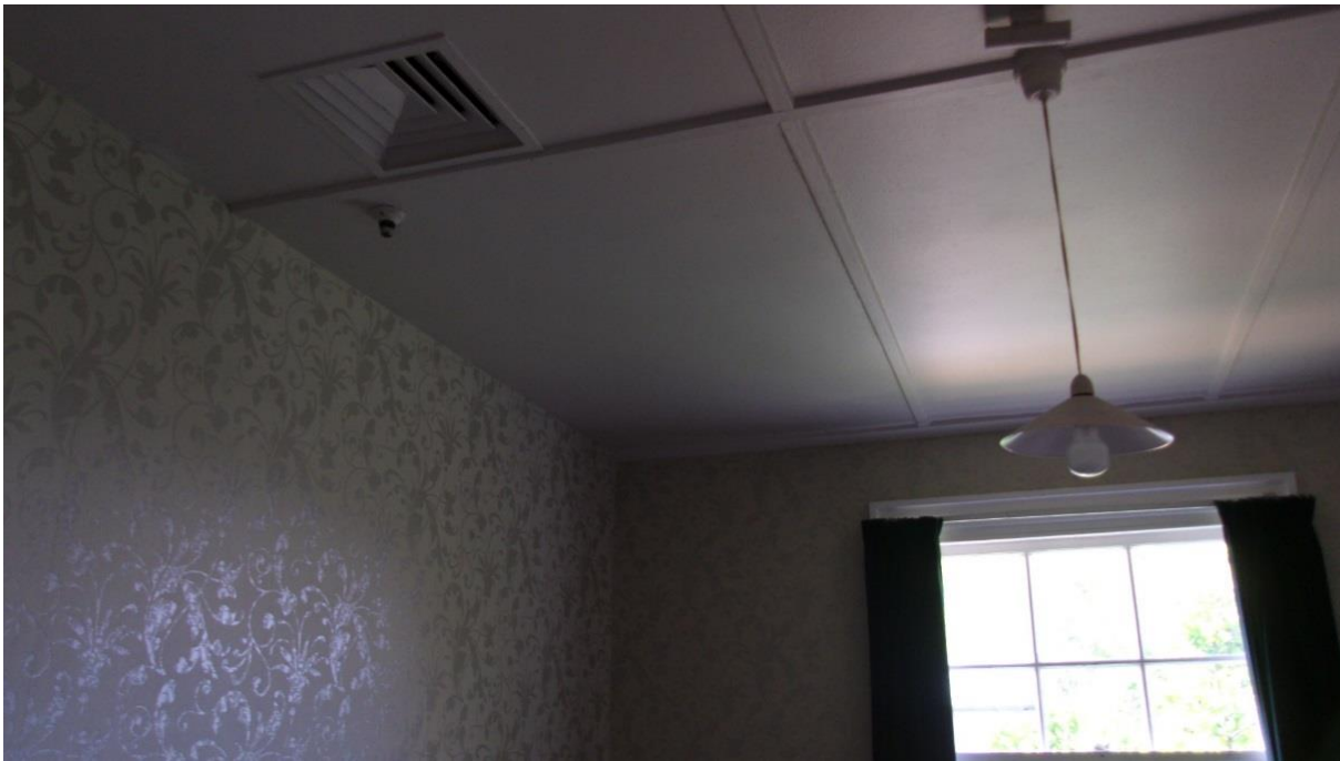
Photo 11. Bedroom in south-west wing with Pinex soft board lined walls and ceiling.
