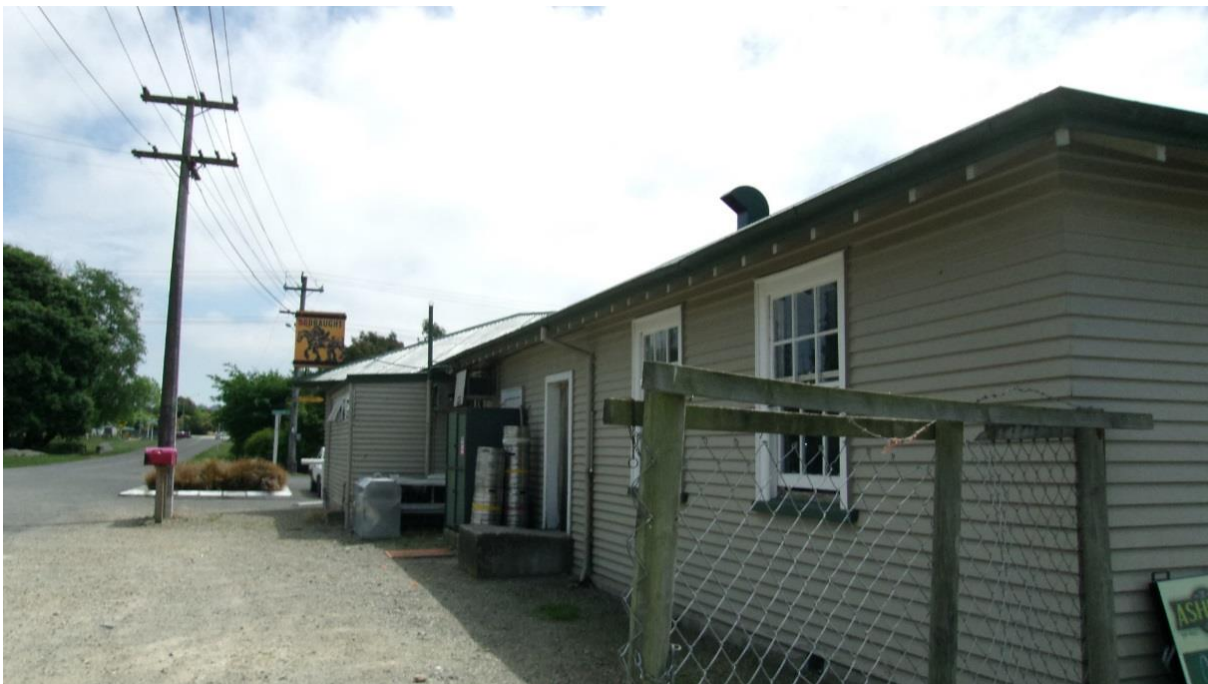
Photo 2. South-west elevation from High Street. Note double hung sash windows indicating pre 1920 construction.
