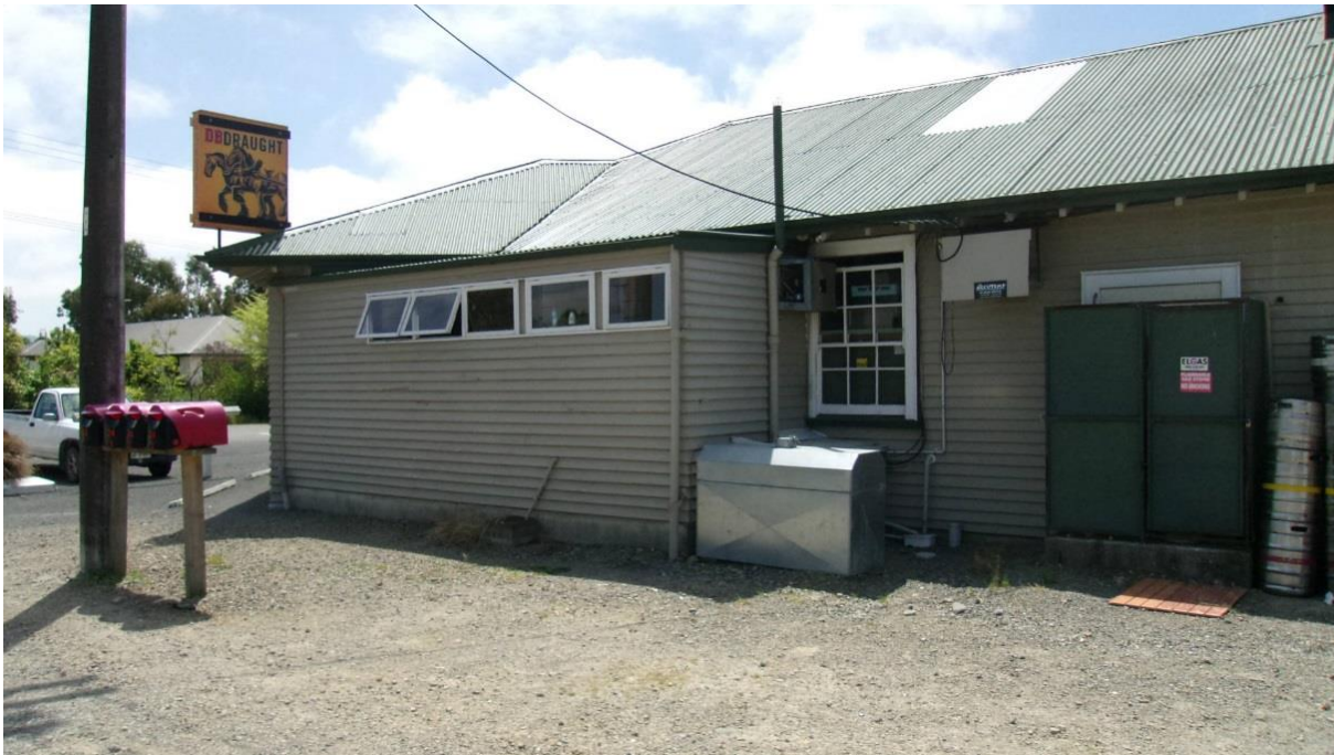
Photo 5. Lean-to extension south-west side for men's toilets. Kitchen at right.
