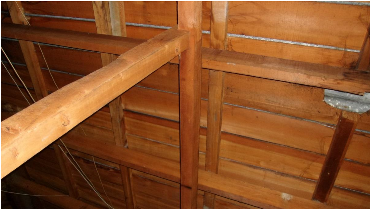
Photo 9. Timber planked sarking and framing to roof.
