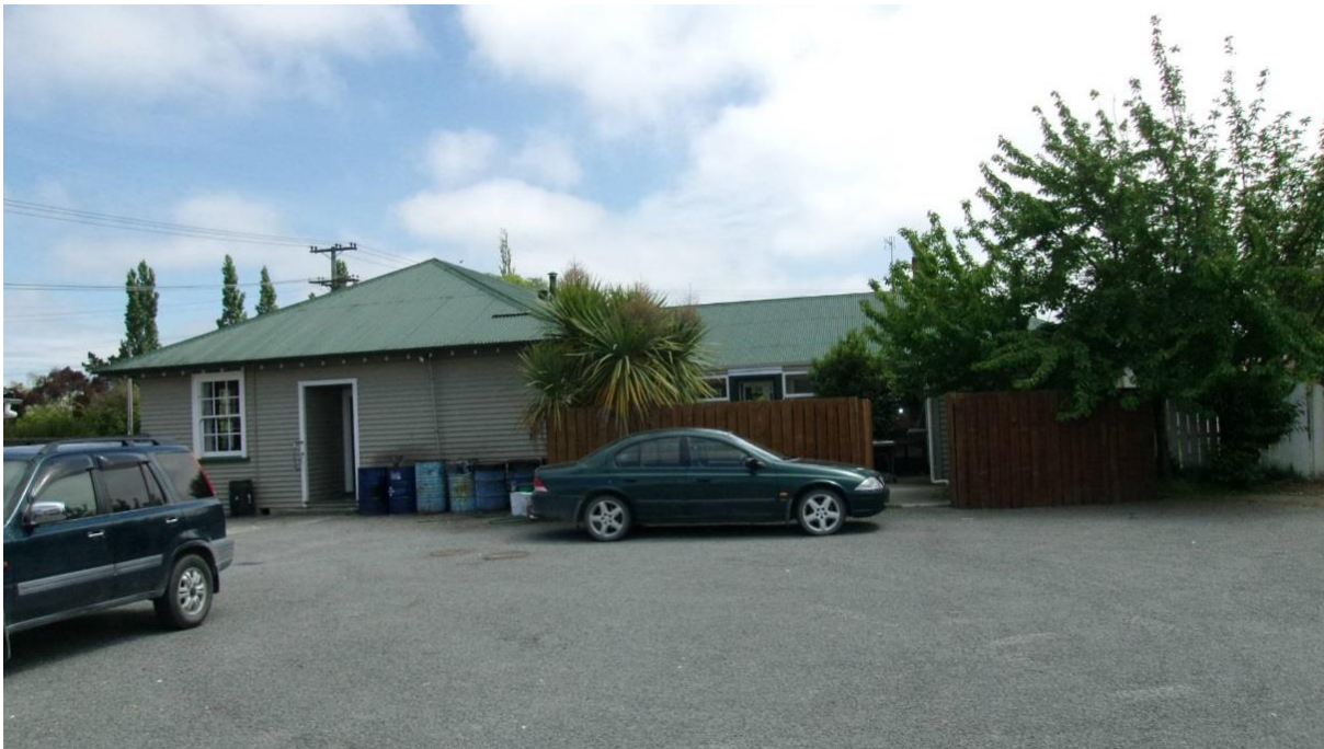
Photo 3. Rear south-east elevation from car park. Public accommodation wing at left. Managers accommodation wing at right behind tree.
