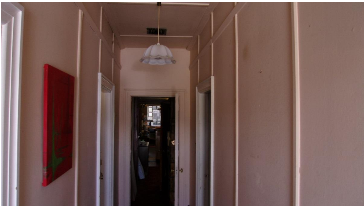
Photo 10. Passageway central in south-west side public accommodation wing. Pinex soft board lined walls and ceiling.
