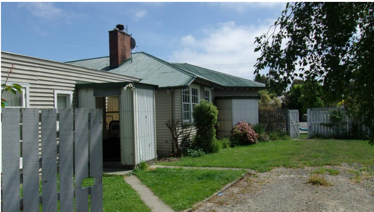
Photo 4. North-east elevation. Private residence part of building including extension, possibly 1967, at left. Note double brick chimney non-functioning.
