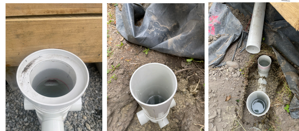
Sewer and Stormwater drains leak tested via Hydrostatic water test to comply with the requirements of G13/AS1 and AS2.
