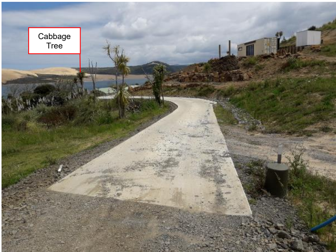
Photo 1 – View of ROW 1 from CH 121 looking back to CH 60.
