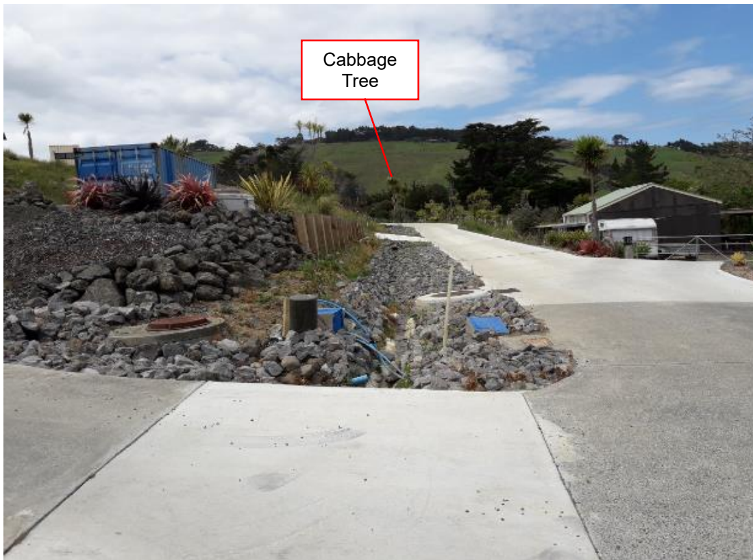
Photo 2 – View of ROW 1 from CH 00 – CH 60
