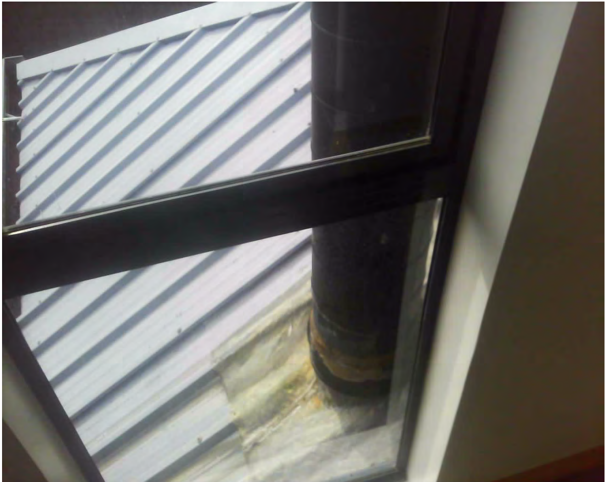
Existing flue flashing Taken at 12:02 PM on Friday 29/04/2016
