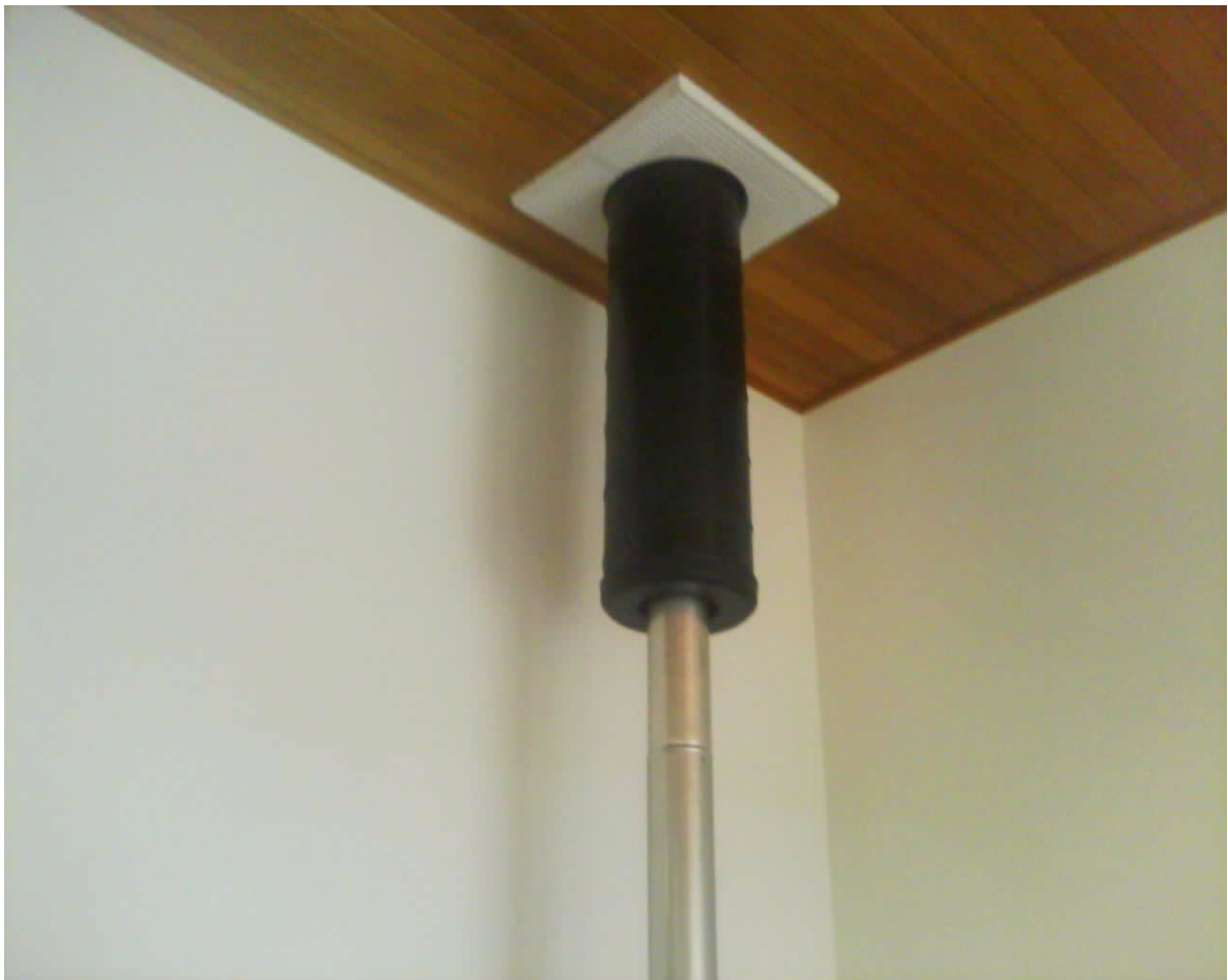
flue entering roof Space Taken at 11:57 AM on Friday 29/04/2016
