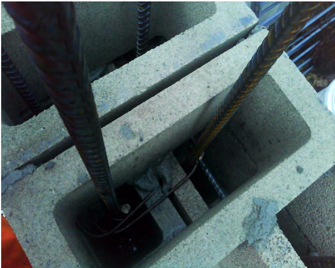
4x HD16s to post, HD16's at 400mm centres horizontally Taken at 10:52 AM on Friday 19/06/2015
