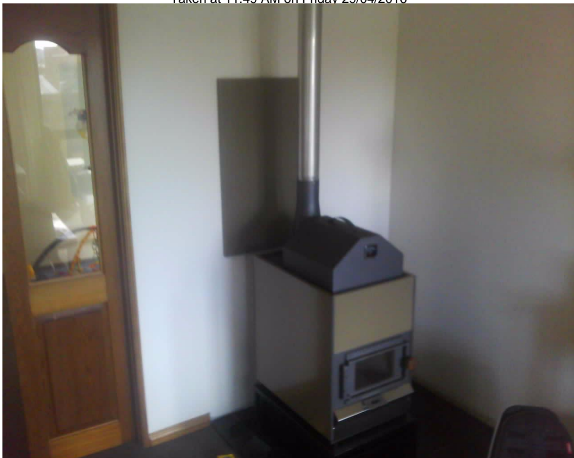
free Standing fire, back panel Installed as fire back is Within 300 mm'
