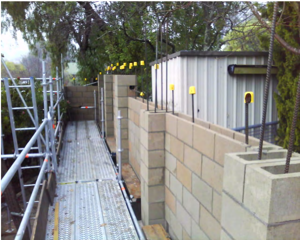
HD12's at 600mm centres main wall 400mm centres to wing walls, area of inspection. Taken at 10:52 AM on Friday 19/06/2015
