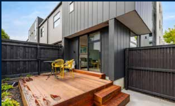
BARBADOES STREET, CHRISTCHURCH CENTRAL
