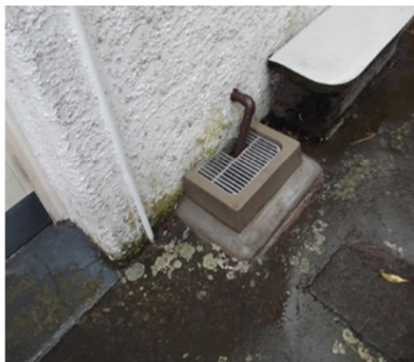
Before and after photos of a low lying gully trap defect that is upgraded to prevent rainwater inflow to the wastewater network.
