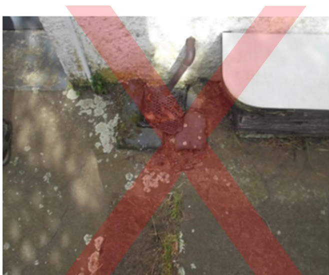
Before and after photos of a low lying gully trap defect that is upgraded to prevent rainwater inflow to the wastewater network.
