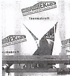
On arrival of doors and windows, cut the COVERIEK403 at each opening on a 45° angle away from each corner. Pull the COVERIEK403 flaps inside and fasten to inside of frame.
