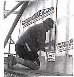
Application of Thermakraft Stud Strap for cavity construction where studs spaced >450mm.
