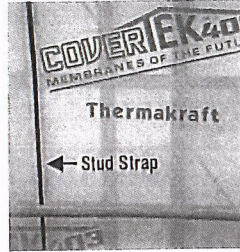
Application of Thermakraft Stud Strap for cavity construction where studs spaced >450mm.
