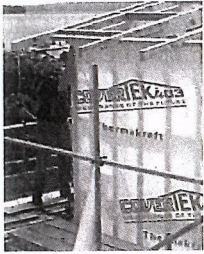
Fix securely to the frame with fasteners such as galvanized 'Little Grippers'.
