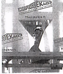
On arrival of doors and windows, cut the COVERIEK403 at each opening on a 45° angle away from each corner. Pull the COVERIEK403 flaps inside and fasten to inside of frame.
