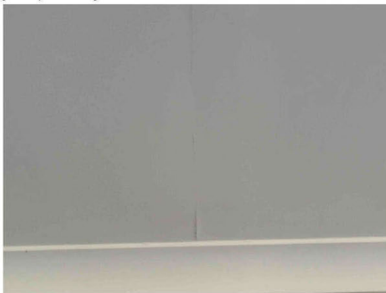
Figure 5 : Ceiling sheet join cracking in the kitchen
