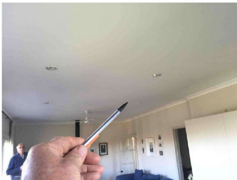
Figure 5 : Ceiling sheet join cracking in the kitchen
