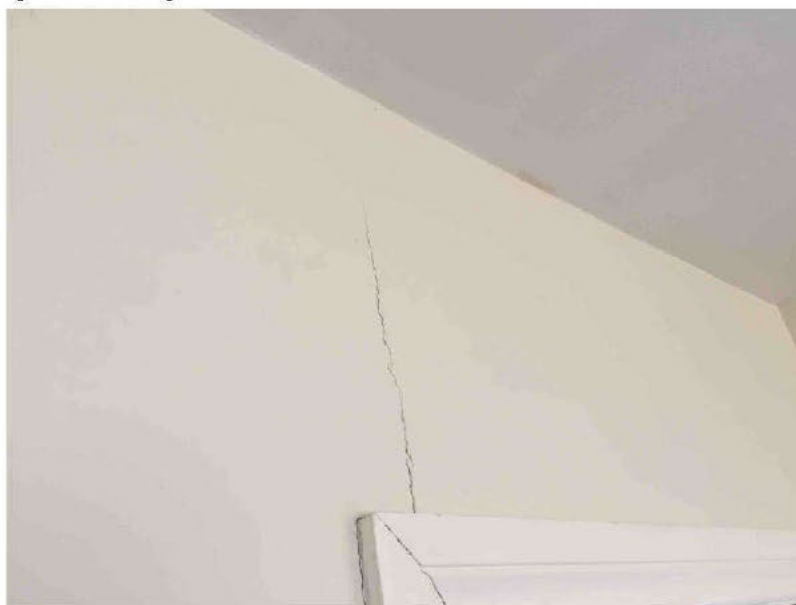
Figure 9 : Pointing to the cracking on office wall
