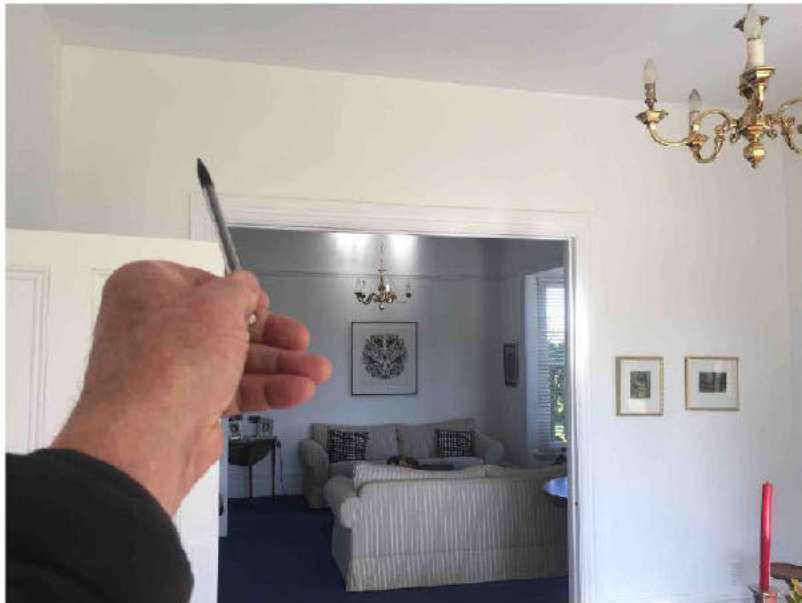
Figure 13 : Pointing to the wall crack above the opening
