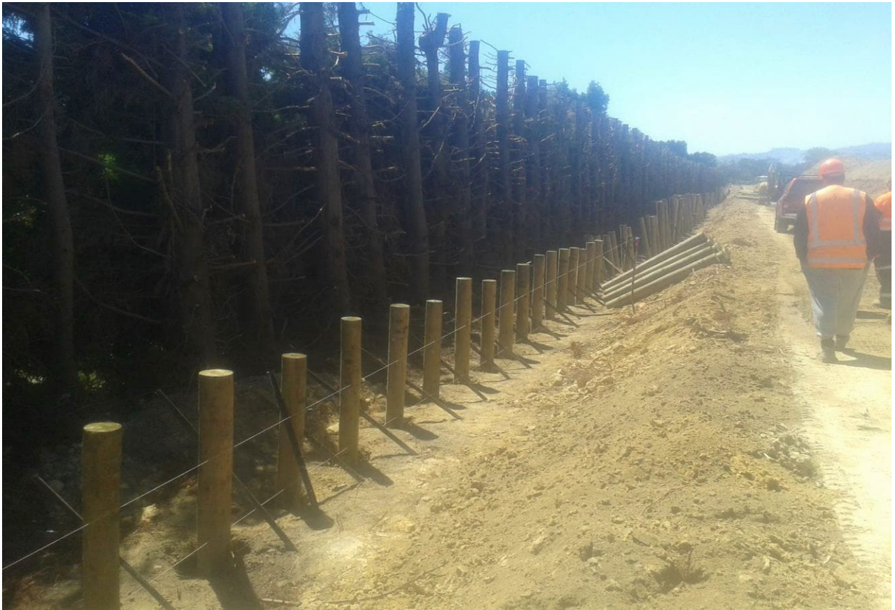
Photograph 3: Photo taken on the 22/11/16 of the final placement and alignment of retaining wall piles.
