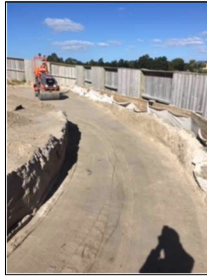
Photo 5: Fill re-compaction
