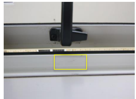
Note these photo examples of the missing window latch receivers
