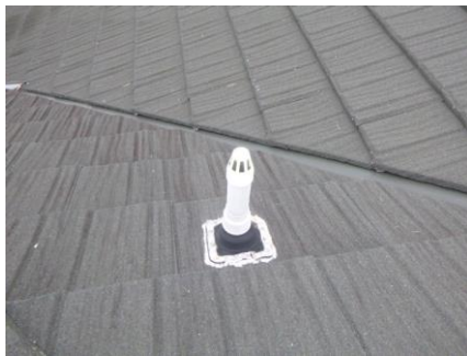
The terminal vent pipes are bird proofed as required
