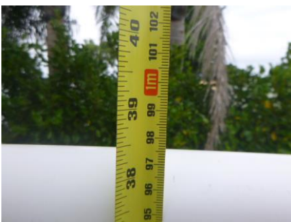
Note that the western handrails are not currently in compliance
