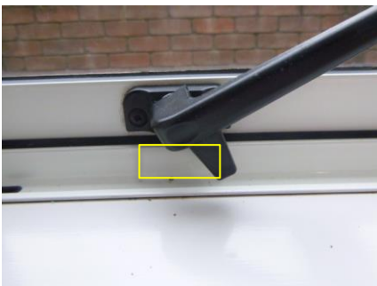
Note these photo examples of the missing window latch receivers
