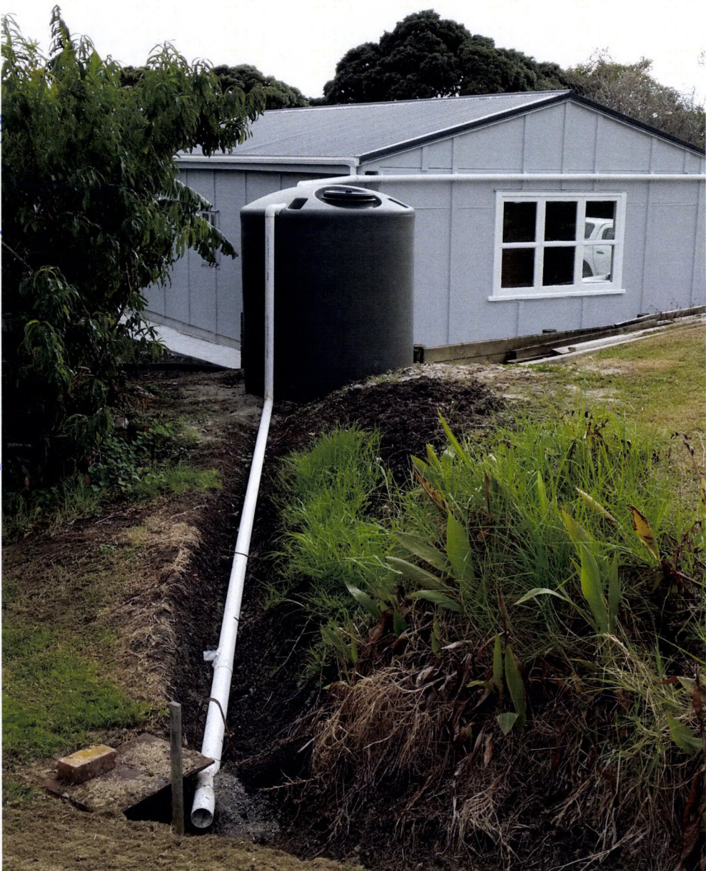
Over flow to SW Drain
