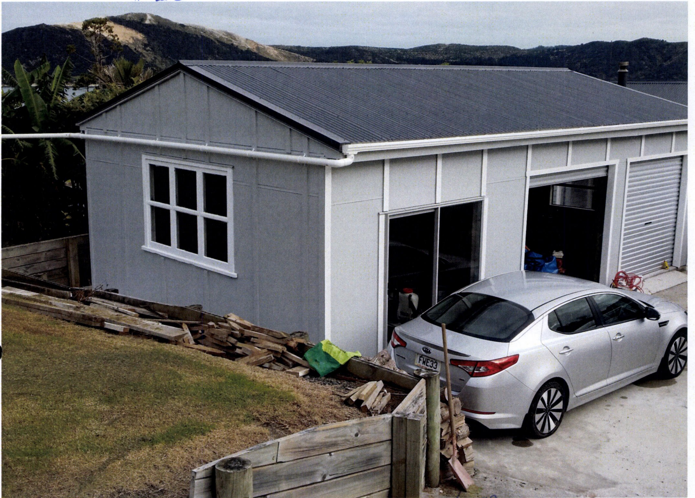
GARAGE DOORS INSTALLED / SPOUTING INSTALLED
