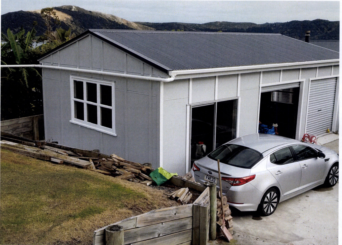
ALL GARAGE DOOR & INSTALLED SPOUTINGS
