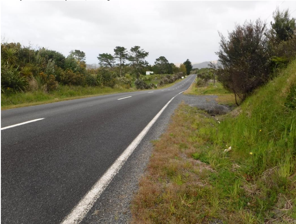
Figure 1 – Site access from Koutu Loop Road, looking south west
