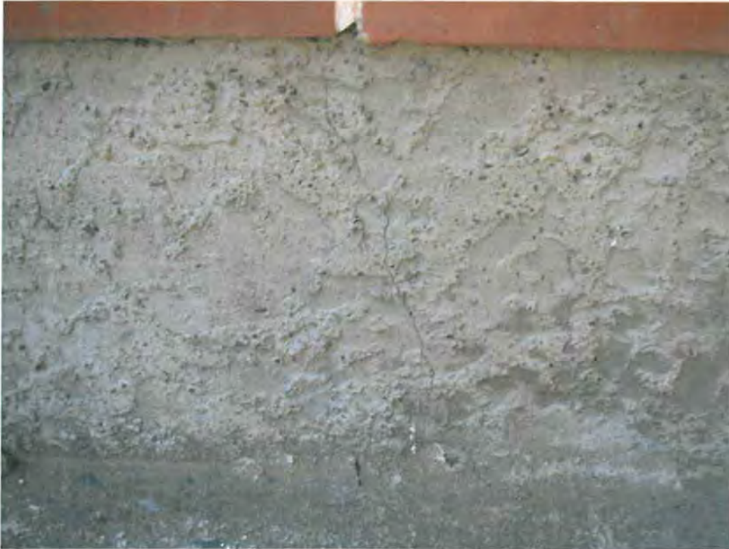
Photo 1: Crack on concrete perimeter foundation wall
