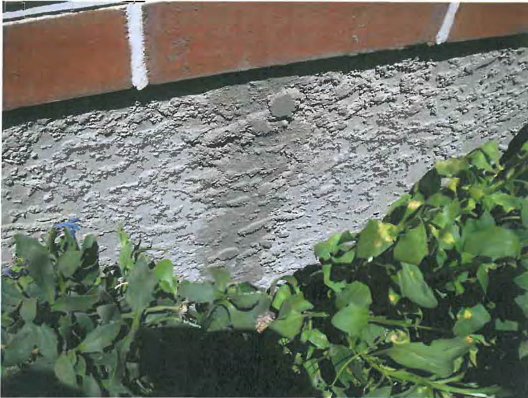
Photo 2: Plaster over repaired crack
