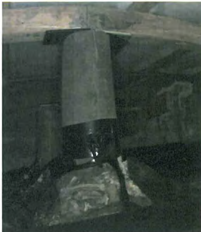
Photo 5: Packer and fixings not as per FEQR detail
