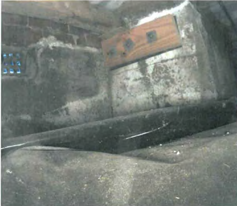
Photo 4: Packer not fixed to bearer and bearer supported by wall plate
