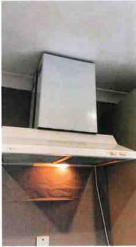
Rangehood: Condition Working
