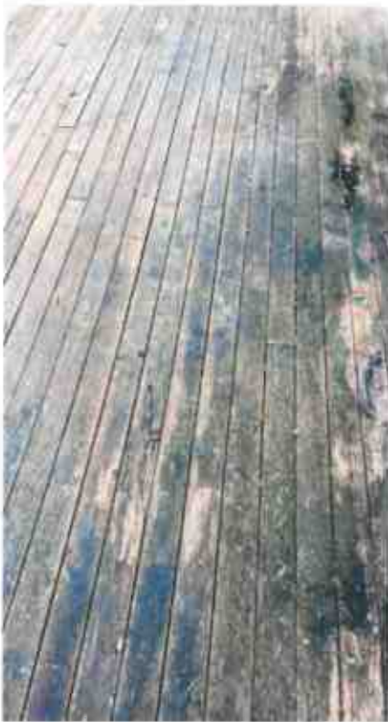
Decking: Material Timber
