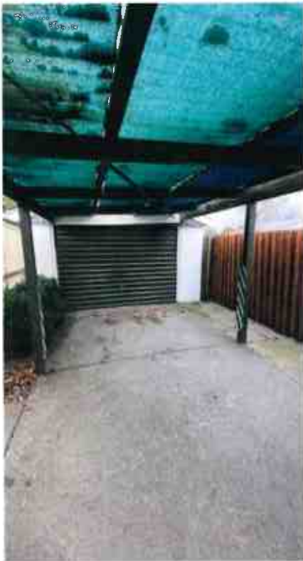
Carport: Garage Exterior Overview Photo
