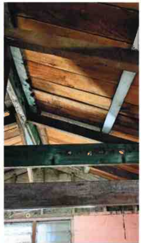
Ceilings: Material Unlined
