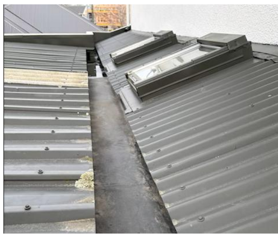
Internal gutter
