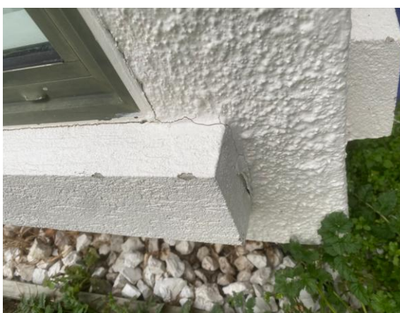
Minor cracking/ potential moisture ingress points to cladding.
