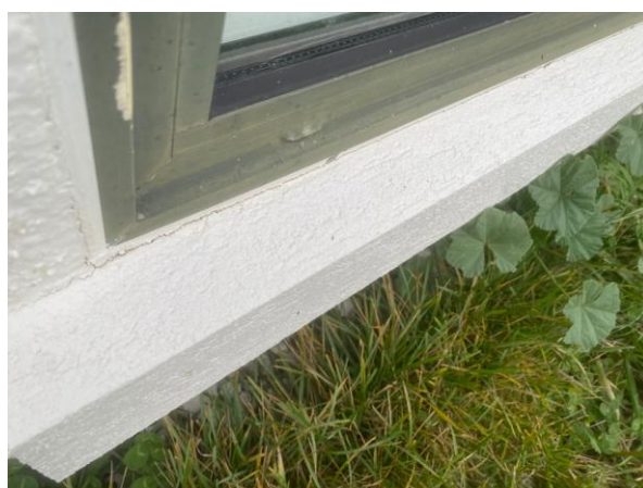
Minor cracking/ potential moisture ingress points to cladding.
