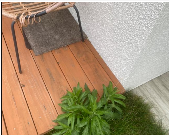
Deck hard against cladding
